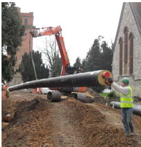
UK Heat Network Installation Galliford Try
